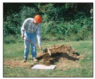
Make sure the cover is on when filling around the enclosure (3.01).
