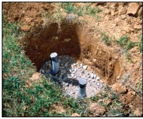
Excavate 6 inches deeper than the depth of the enclosure and add 6 to 8 inches of gravel or crushed rock (1.02).
