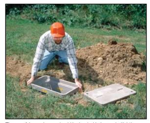
The top of the enclosure should be level with the grade (2.01).
